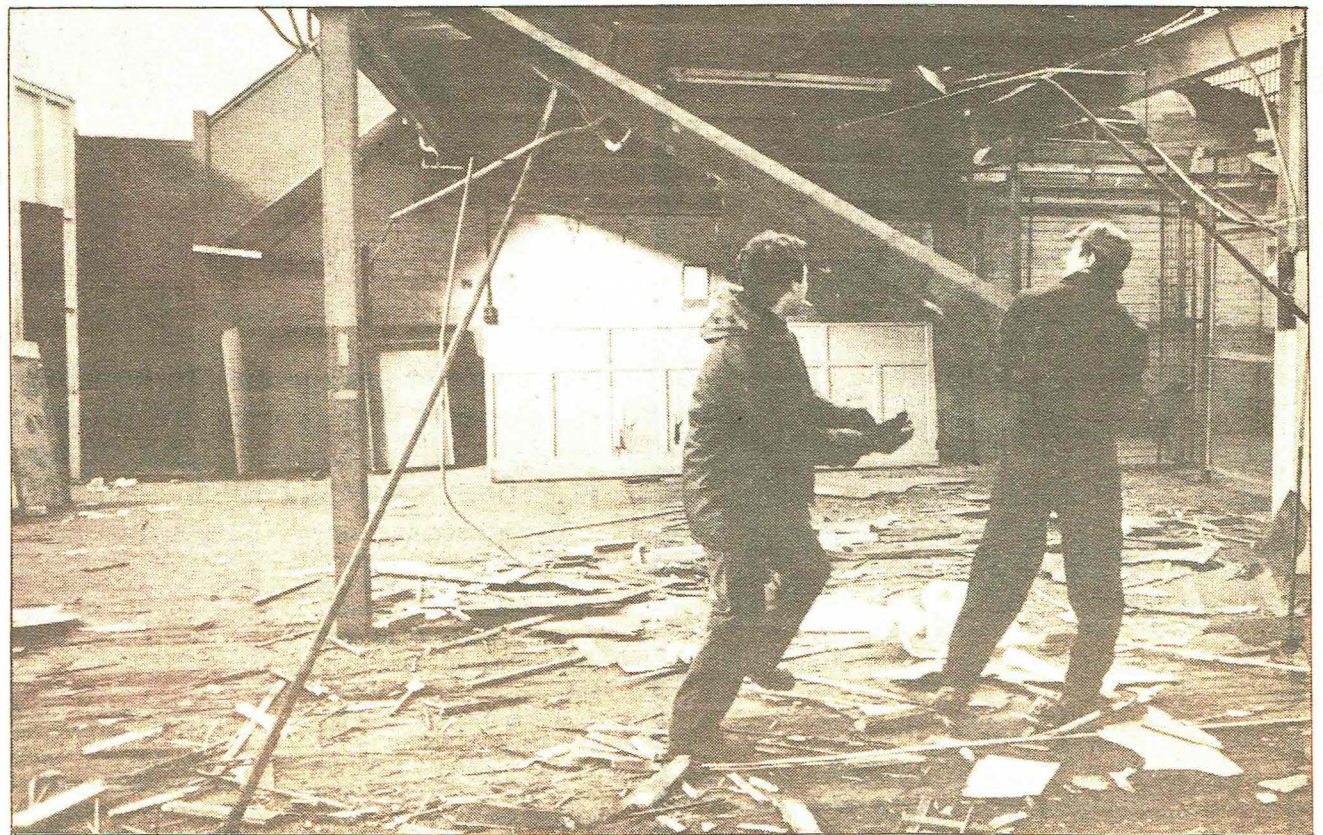
Manpower Service Commission workers dismantling Leyland South works this month. They are taking the wooden floor beams to renovate the out-building of a stately home. Photo: D Doran
